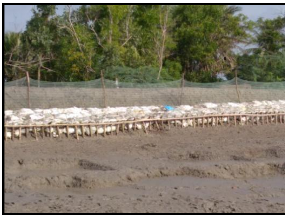
Fig14: Construction of Embankment
