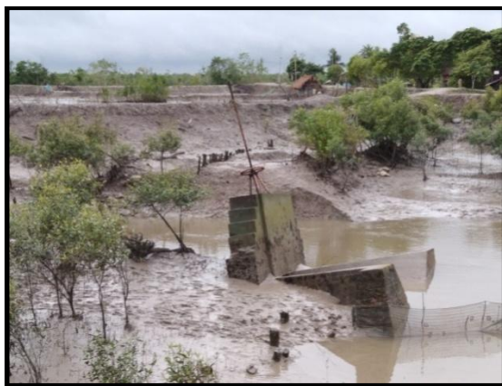
Fig12: Ruined sluice gate
